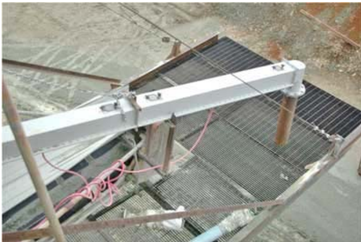
Air slide for filling trucks
